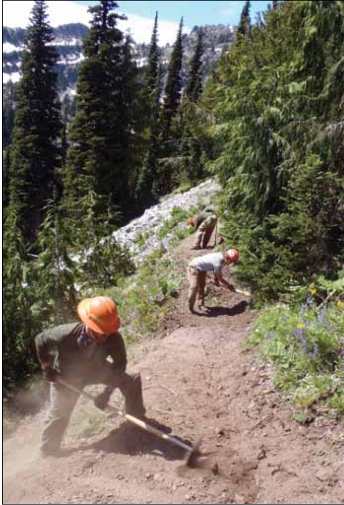
Four Northwest Service Academy AmeriCorps crews worked on the PCT in 2011. This crew reconstructed 3,750 feet of trail tread in the Okanogan-Wenatchee National Forests.
