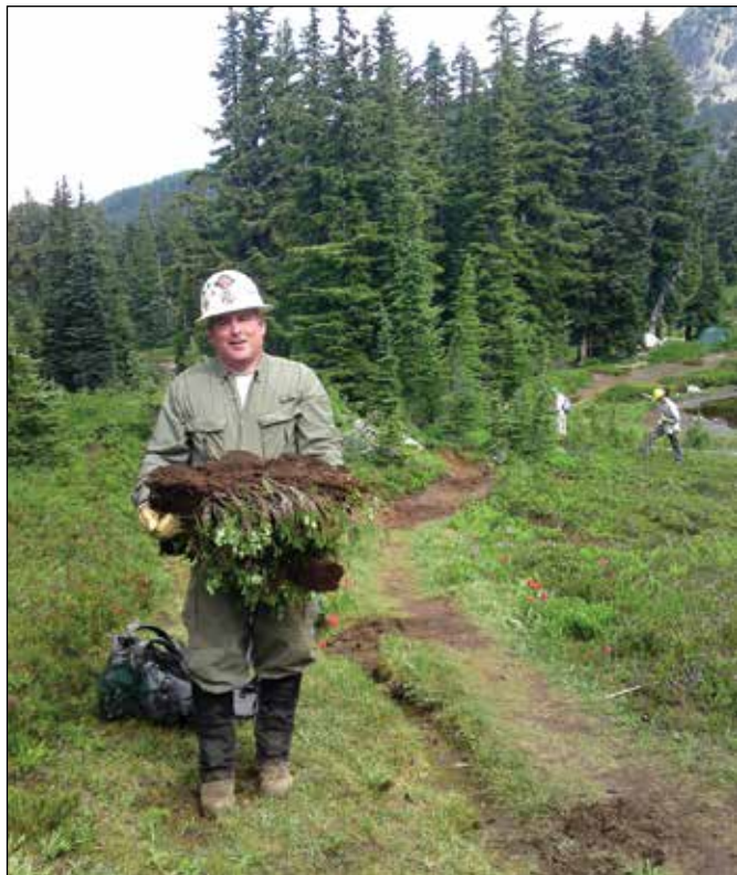
Skyline Crew volunteers carefully transplanted subalpine vegetation in order to close unauthorized user trails.
