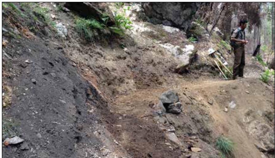
PCTA fielded a corps crew to perform much needed restoration work on the Klamath National Forest in a fire-damaged ecosystem. The crew spent nearly three weeks redigging tread, repairing crucial drainages and building retaining walls to limit further damage to the PCT and erosion run off into the Grider Creek drainage.
