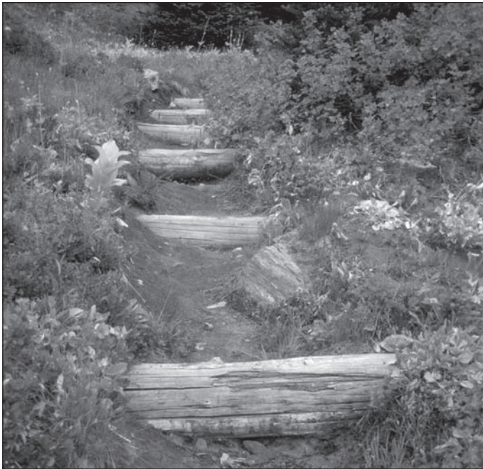
Figure 1. Large check dams, over the years, will help this gully fill in. These check dams need an apron of loose rocks down from each log to prevent water scouring. Scarifying, planting rocks and transplants, adding fill, seeds, and debris will speed the process. (IMAGE COURTESY OF THE USFS)
