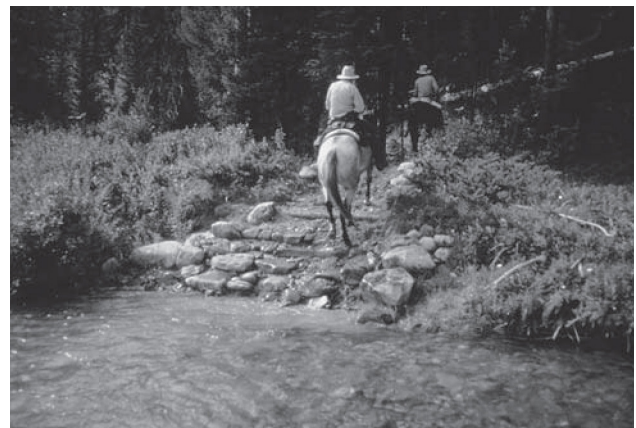
Figure 2. Fords should be established in a straight and shallow section of a stream. Approaches must climb above the high-water line to prevent water from running down the trail. Note the armored entrance/exit ramp into the ford, constructed of rock and gravel. (IMAGE COURTESY OF THE USFS)
