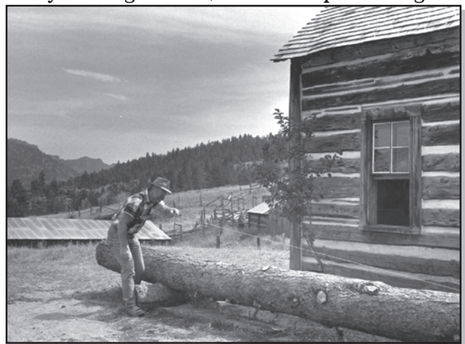
Figure 99—The chalk line will mark the top side of the hewn surface.
