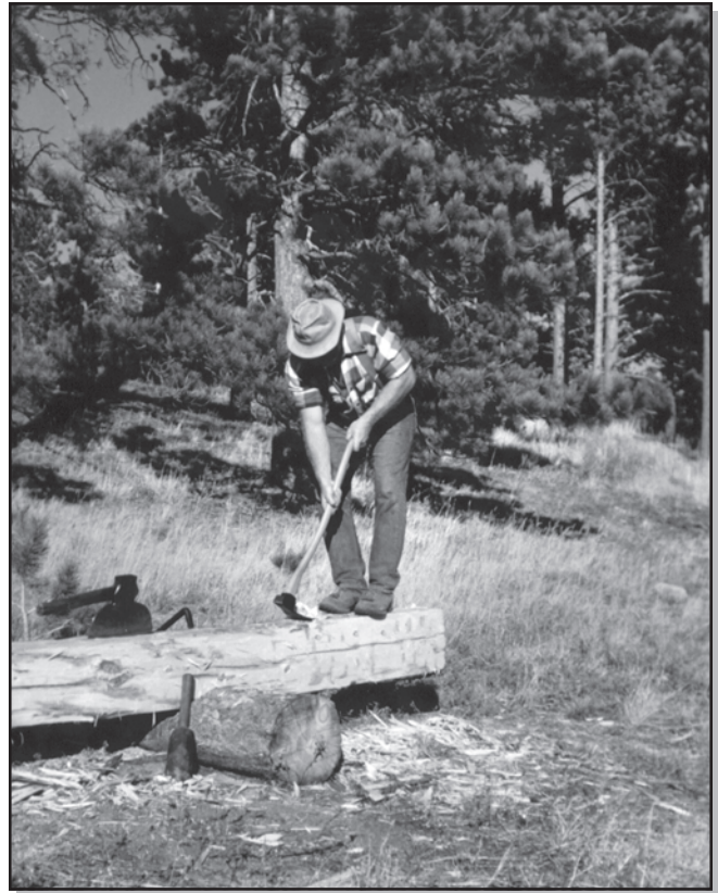
Figure 104—Adz work requires the utmost concentration to avoid cutting your feet.
