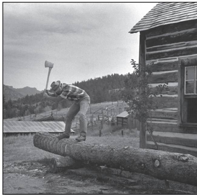
Figure 101—In the scoring technique called juggling, you cut a shallow V-notch down to the depth of the chalk line. Slash scoring is a different technique that doesn't involve cutting a V-notch.
