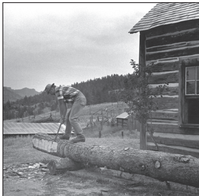
Figure 102—Finish the juggling process by removing the excess wood between V-notches with a single-bit ax.
