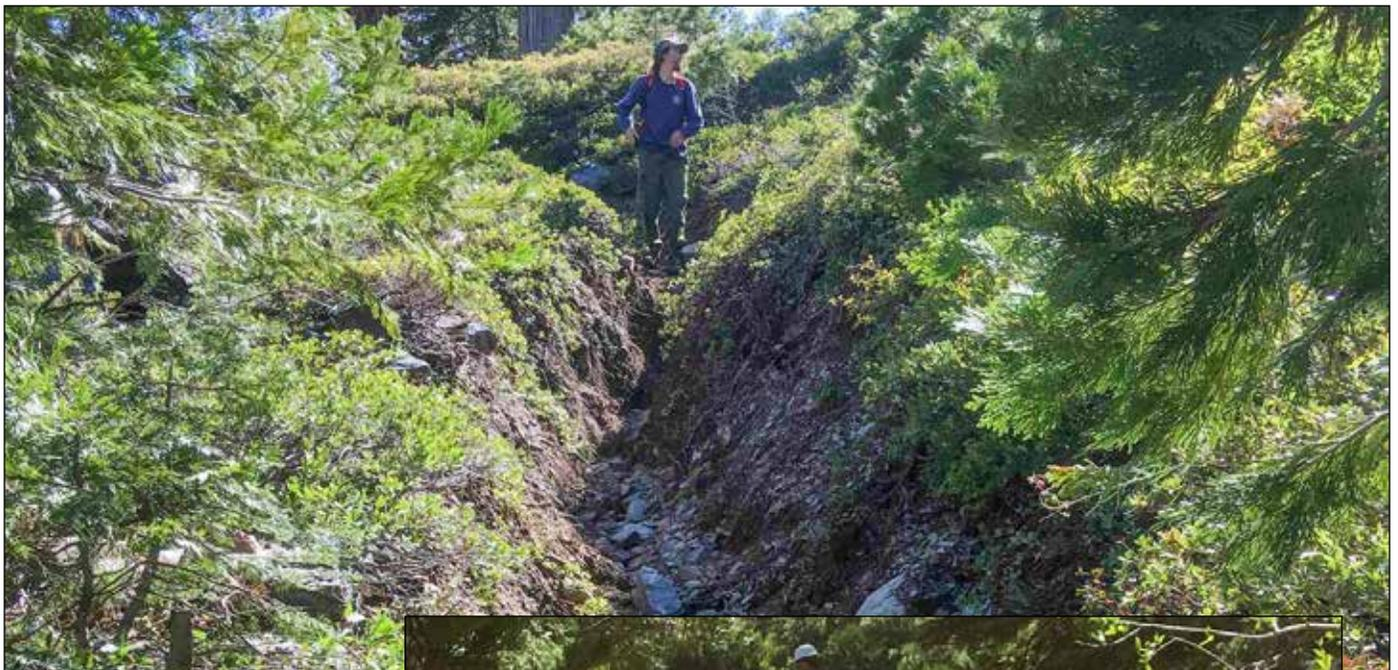
*On the Lassen National Forest Almanor Ranger District, a drainage had shifted out of its channel causing significant erosion and scouring material out of the trail leaving the PCT no longer safe with a deep trench with a steep five-foot drop-off. In 2017, American Conservation Experience corps crews spent 808 hours reconstructing the PCT in this area. Thanks to this effort, the PCT is up to trail standards, but most importantly it is now safely passable for hikers and horseback riders.*
