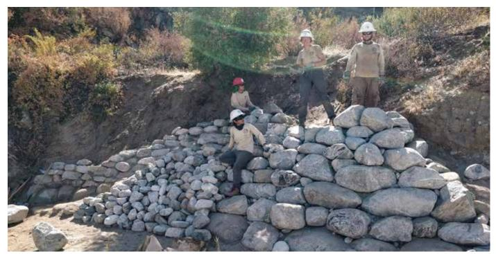
Just outside of Palm Springs, California, ACE crew members quarry and place rock by hand on the stone staircase they are building so the public can access the PCT.
