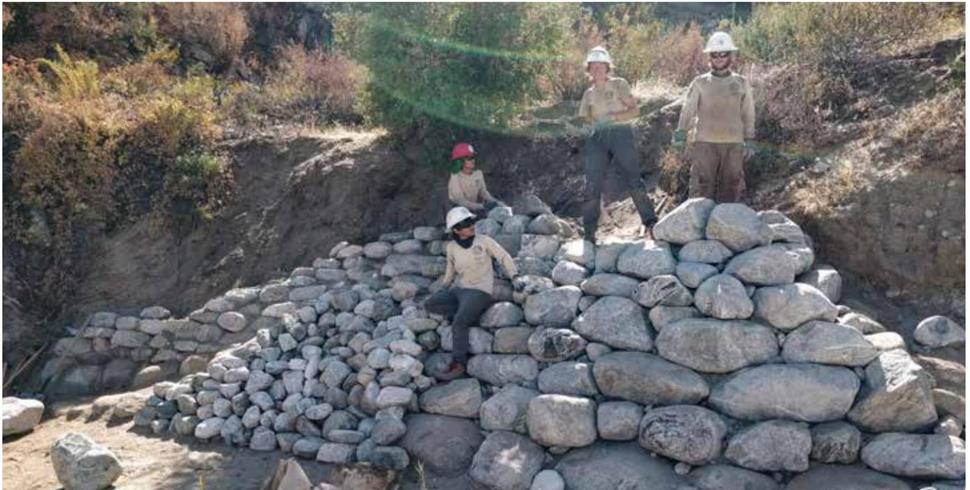
*Just outside of Palm Springs, California, ACE crew members quarry and place rock by hand on the stone staircase they are building so the public can access the PCT.*
