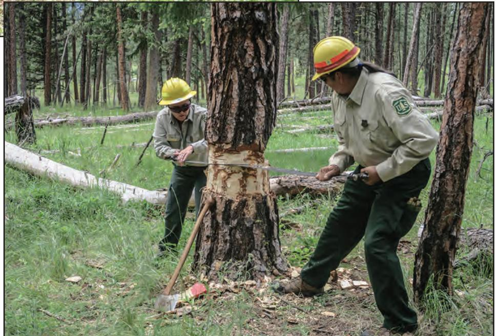
Figure 3-7—Sawyers using a crosscut saw to perform a back cut. Note the ax and wedges at the base of the tree.
