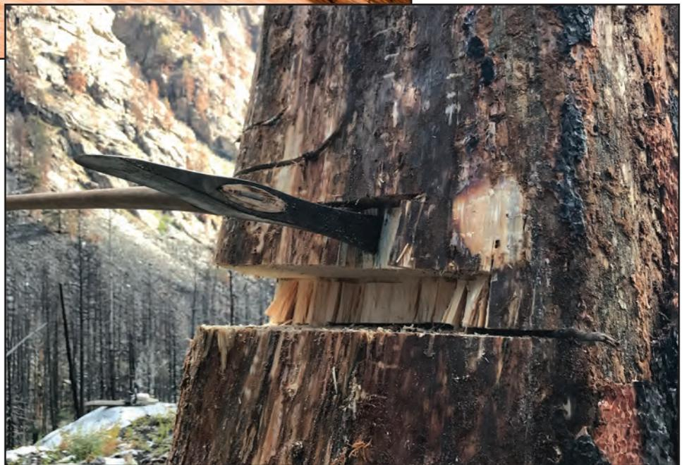
Figure 5-14—Using the chisel end of an undercutter ax between two horizontal cuts to create an undercut.
