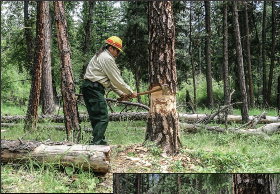
Figure 3-6—An axman chopping a sloping cut.
