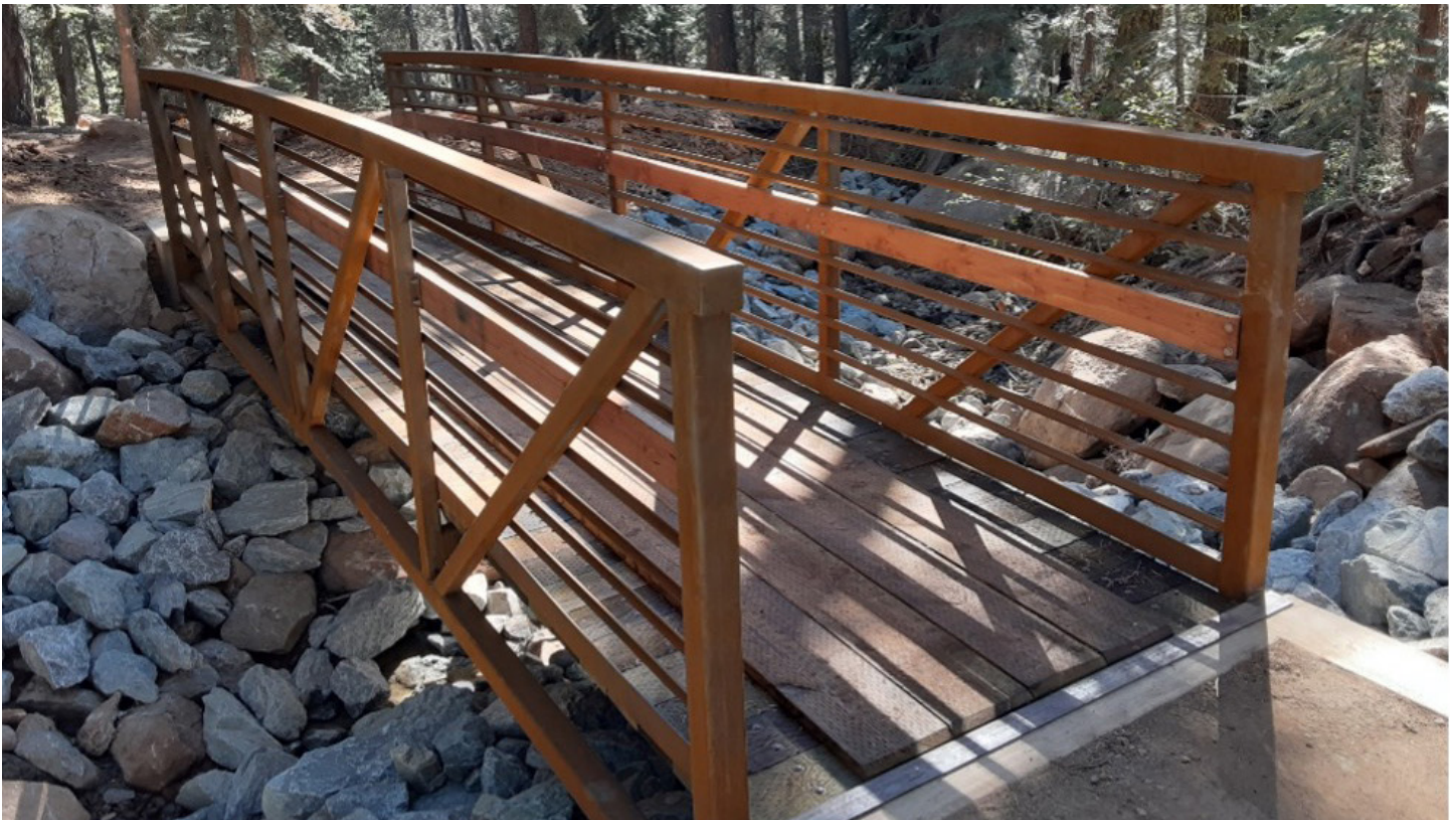
PCT bridge on the Eldorado National Forest near Echo Lakes. The bridge was installed in October prior to the winter weather conditions. Additional work was done to armor and protect the concrete bridge abutments and banks of the creek.
